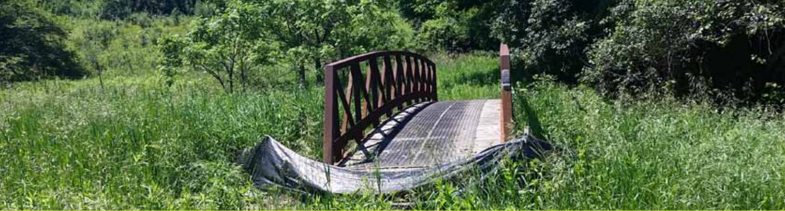
The new bridge at Cruickston Creek. Photo by C. Pope
